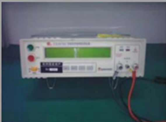
Insulation resistance test
